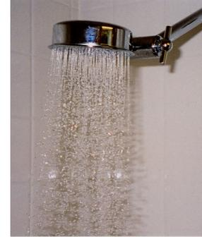
When the distance between the hot water tap and the shower cap is too long it introduces an excessive delay. This may give rise to growing oscillations in temperature resulting from the user lack of understanding of the situation
